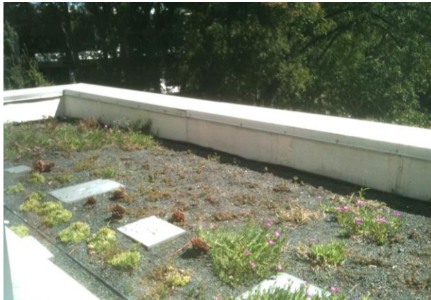
Green Roof – Robert C. Wilson Pharmacy Building
