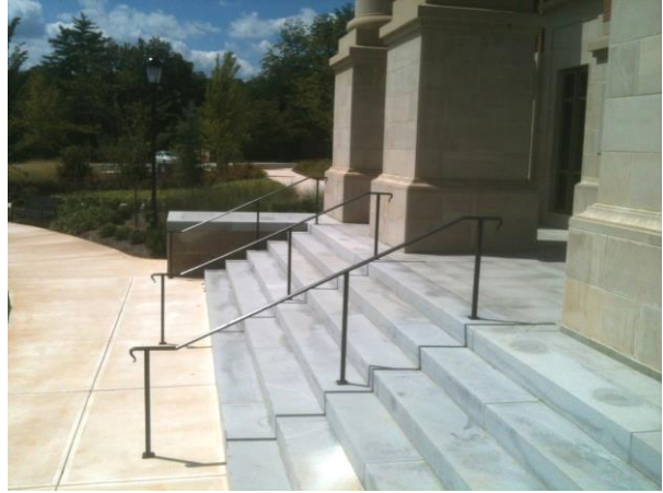
Stairs & Handrails – Special Collections Library
