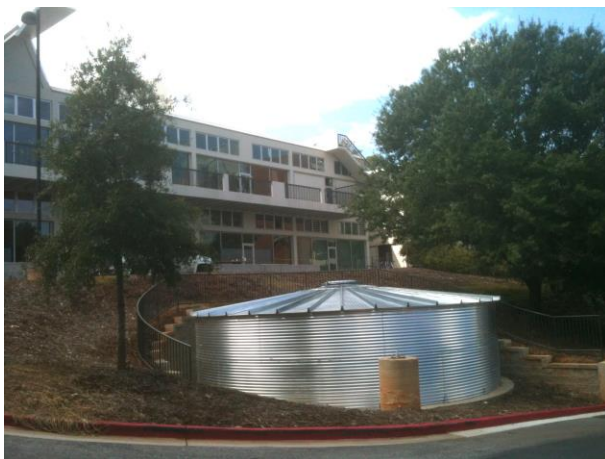
Above-Ground Cistern – Jackson Street Building
