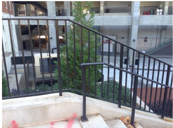
Handrails & Adjacent Guardrail – Reed Plaza
