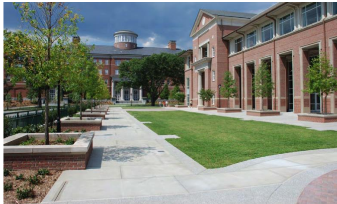
Green Roof – Tate Student Center
