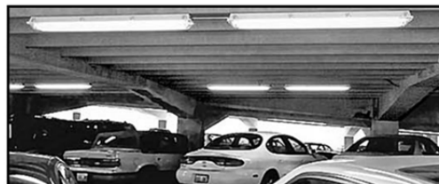
Covered Parking Structure - Up to -20° F starting
