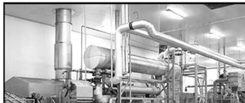
Potato Chip Manufacturing Facility
