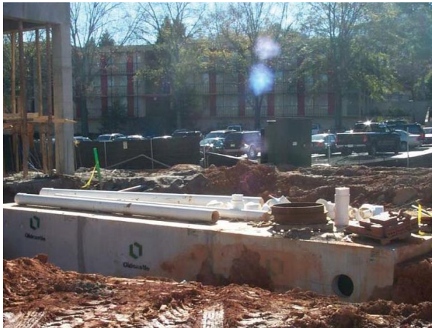
Underground Cistern – Paul D. Coverdell Center
