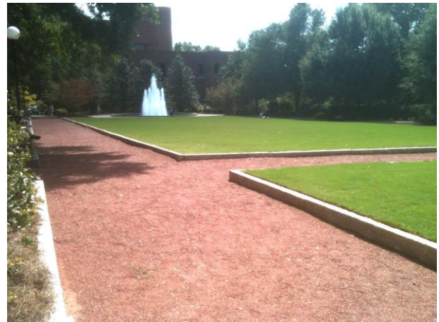
Granular Paving – Herty Field
