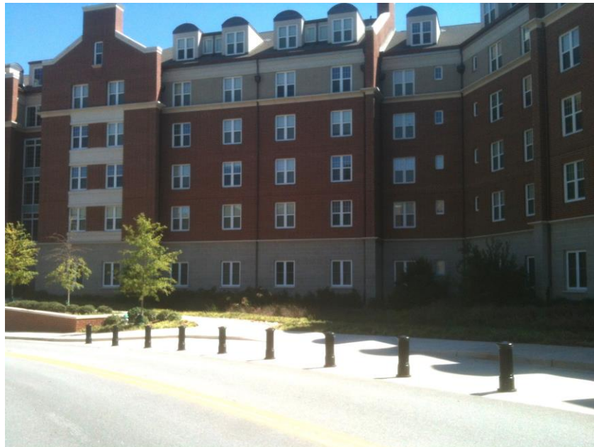
Security Bollards – Building 1516
