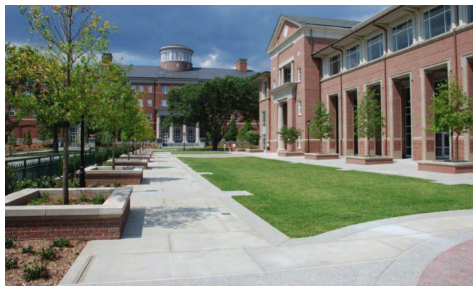
Green Roof – Tate Student Center
