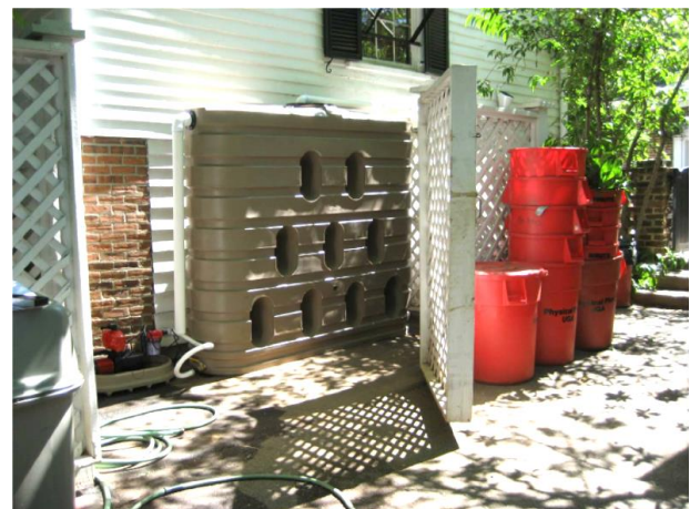
Above-Ground Cistern – Founders House
