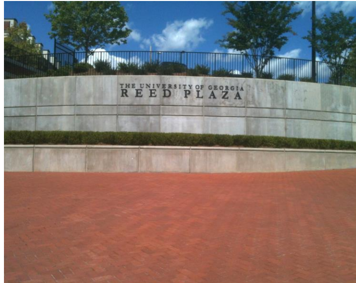
Brick Work – Reed Plaza
