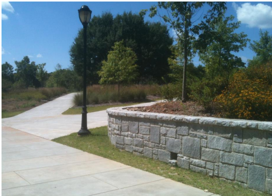
Granite Rubble Wall – Lamar Dodd School of Art & Georgia Museum of Art
