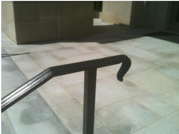
Handrails – Special Collections Library
