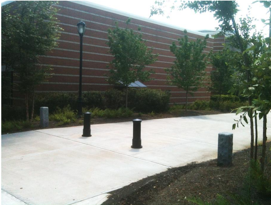
Security Bollards – Hugh Hodgson School of Music & Performing Arts Center
