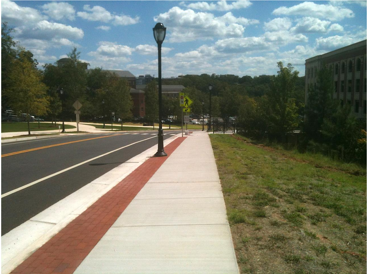
Sidewalk with Brick Accent Banding – Hull Street Deck
