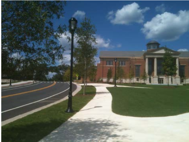
Sidewalk With Landscape Treatment – Special Collections Library
