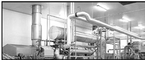
Potato Chip Manufacturing Facility
