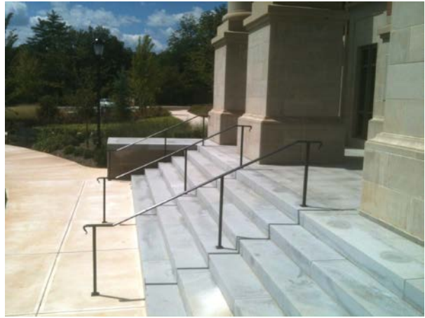
Stairs & Handrails – Special Collections Library
