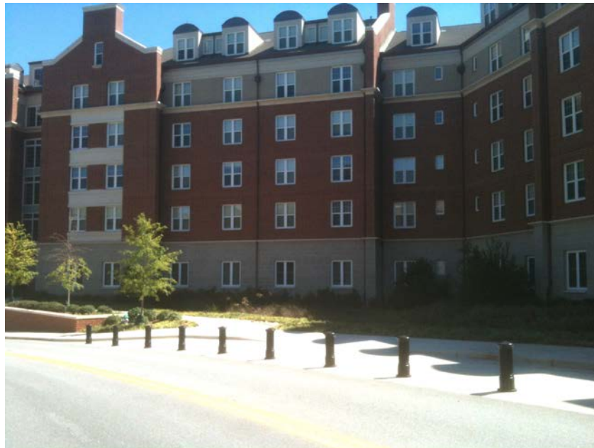
Security Bollards – Building 1516
