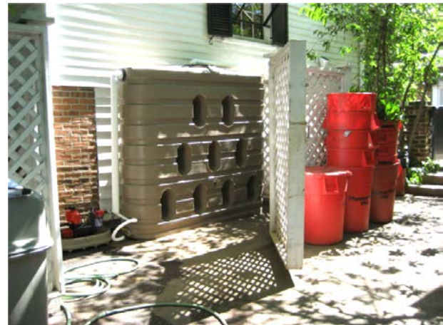
Above-Ground Cistern – Founders House
