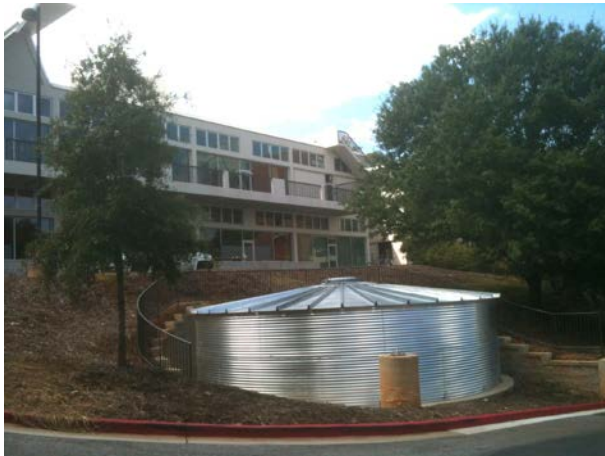
Above-Ground Cistern – Jackson Street Building
