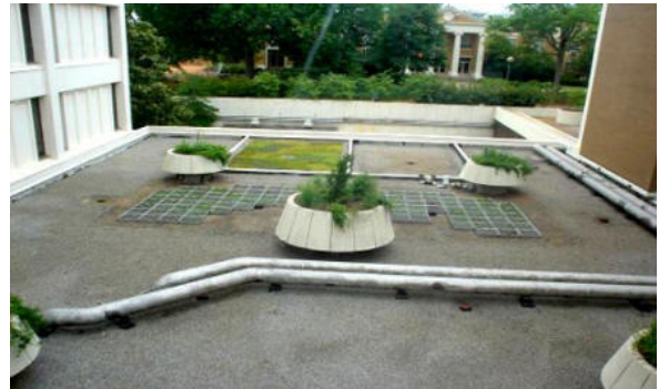
Green Roof – Science Library
