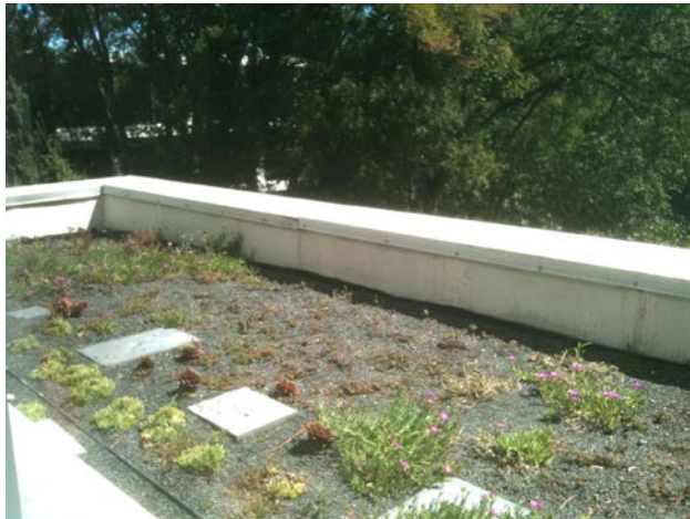
Green Roof – Robert C. Wilson Pharmacy Building
