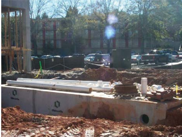
Underground Cistern – Paul D. Coverdell Center
