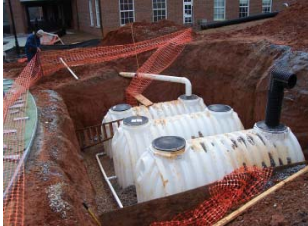
Underground Cistern – Miller Learning Center
