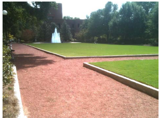
Granular Paving – Herty Field
