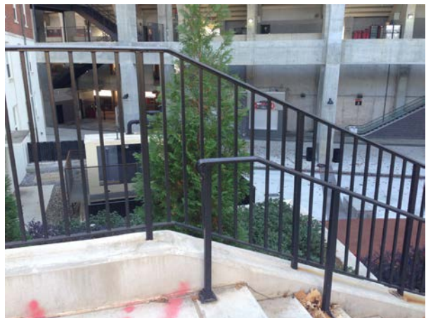
Handrails & Adjacent Guardrail – Reed Plaza
