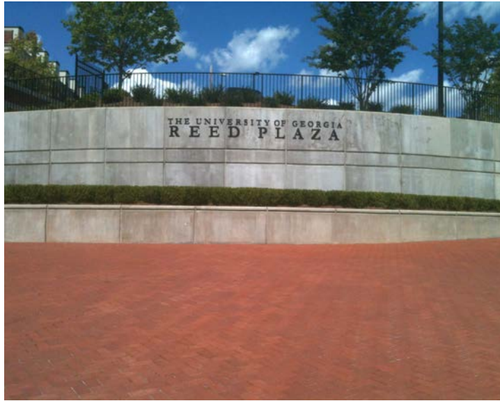
Brick Work – Reed Plaza
