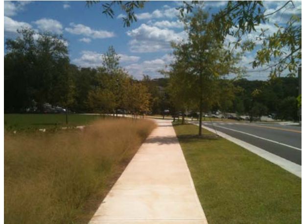
Sidewalk With Landscape Treatment – Special Collections Library
