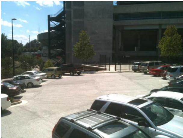
Porous Paving Parking Lot – Reed Plaza
