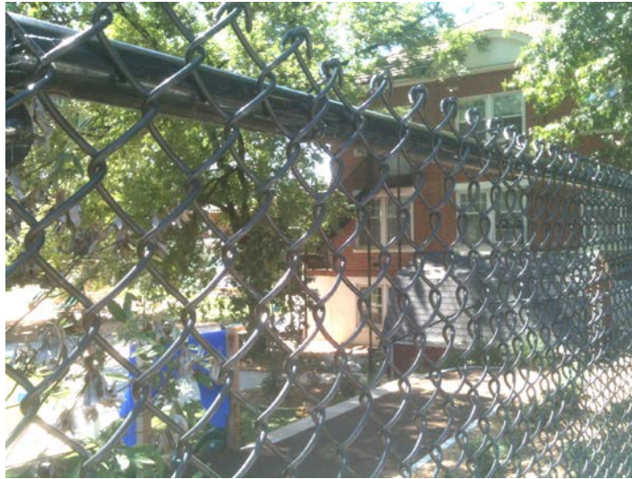
Chain-Link Fence – McPhaul Child & Family Development Center
