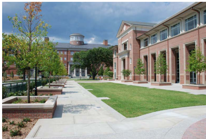
Green Roof – Tate Student Center
