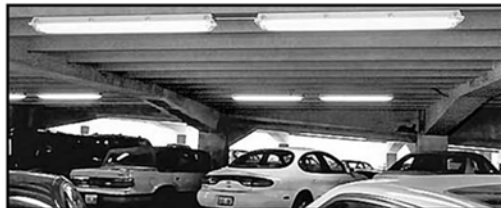
Covered Parking Structure - Up to -20° F starting
