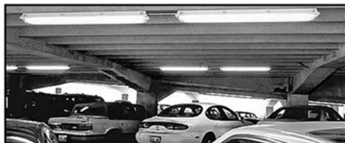
Covered Parking Structure - Up to -20° F starting
