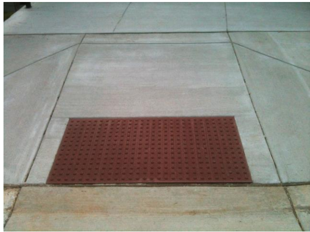
Truncated Domes – Special Collections Library & Hull Street Deck
