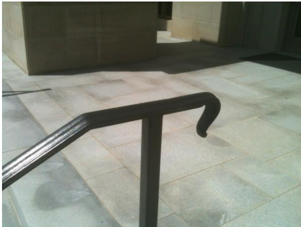
Handrails – Special Collections Library
