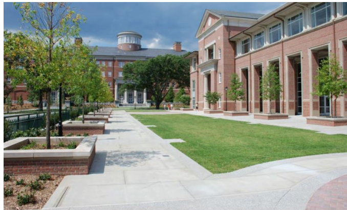
Green Roof – Tate Student Center
