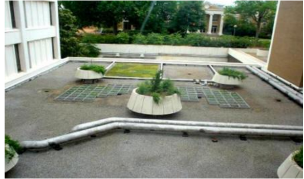
Green Roof – Science Library
