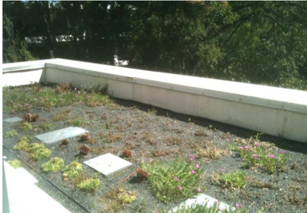
Green Roof – Robert C. Wilson Pharmacy Building
