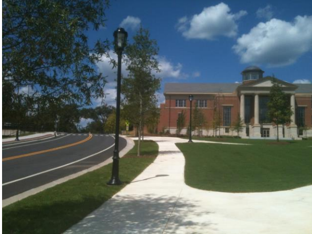
Sidewalk With Landscape Treatment – Special Collections Library
