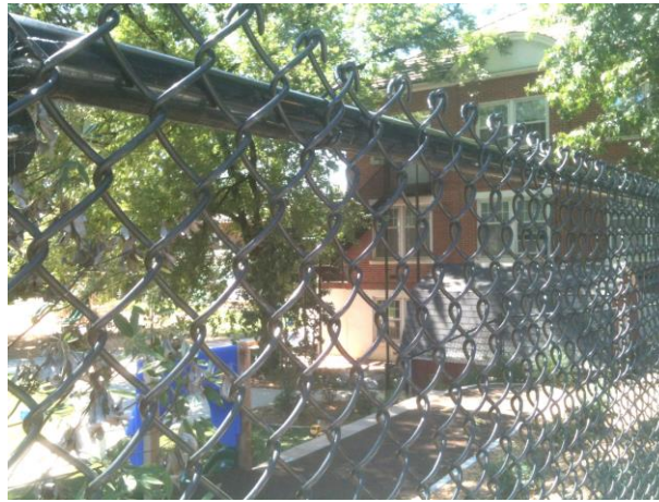
Chain-Link Fence – McPhaul Child & Family Development Center
