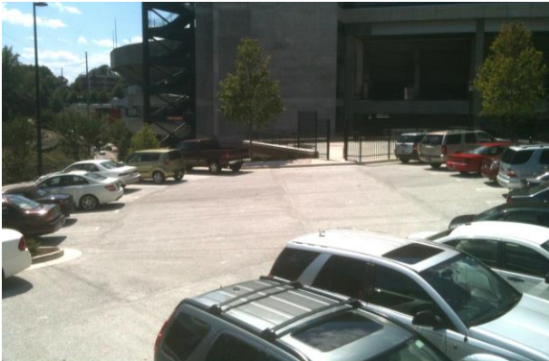
Porous Paving Parking Lot – Reed Plaza
