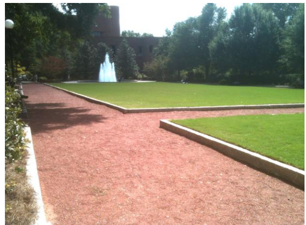
Granular Paving – Herty Field
