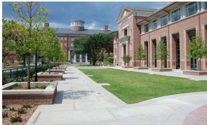
Green Roof – Tate Student Center
