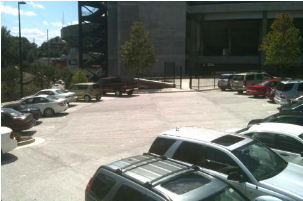
Porous Paving Parking Lot – Reed Plaza
