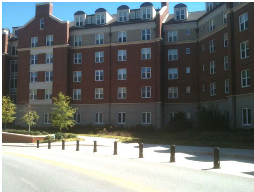
Security Bollards – Building 1516
