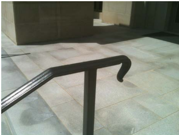
Handrails – Special Collections Library
