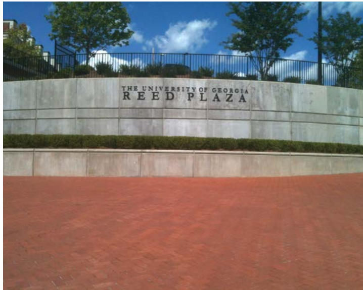
Brick Work – Reed Plaza
