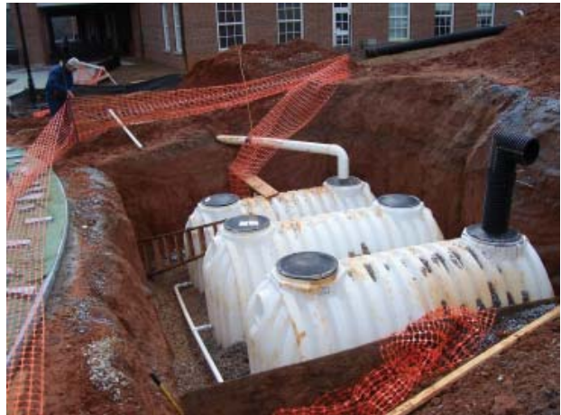
Underground Cistern – Miller Learning Center
