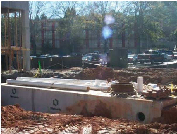
Underground Cistern – Paul D. Coverdell Center
