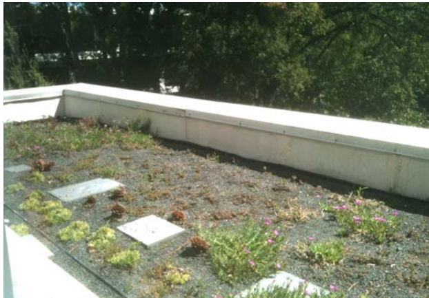
Green Roof – Robert C. Wilson Pharmacy Building
