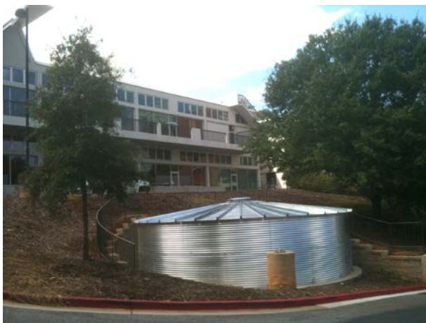
Above-Ground Cistern – Jackson Street Building
