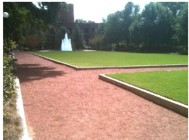
Granular Paving – Herty Field
