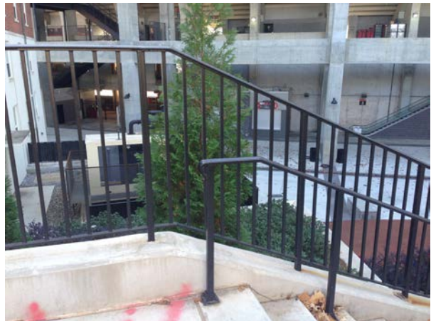
Handrails & Adjacent Guardrail – Reed Plaza
