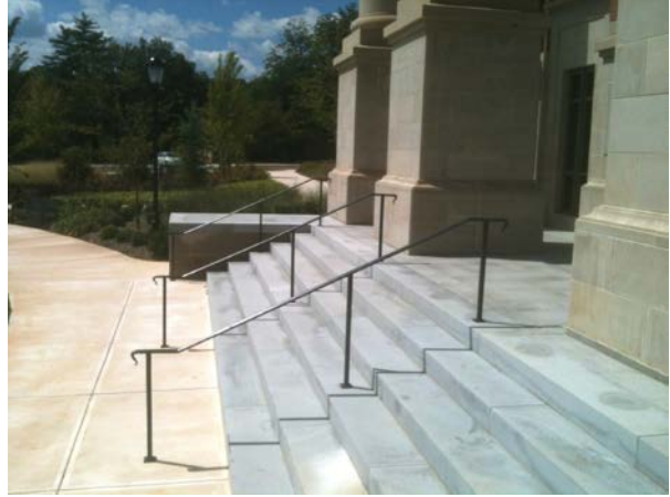
Stairs & Handrails – Special Collections Library
