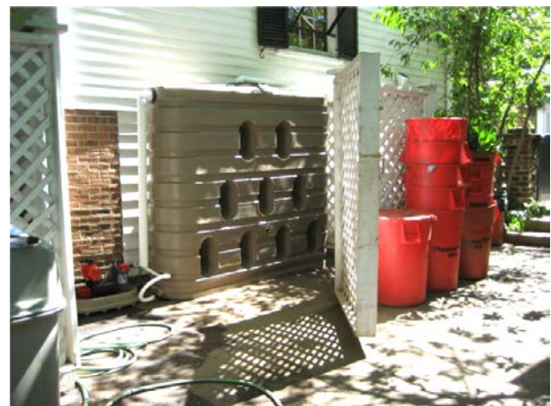
Above-Ground Cistern – Founders House
