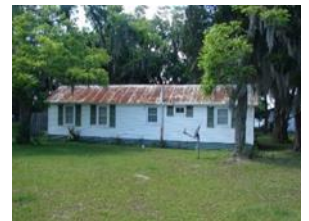
Figure 617. Maintenance Shop 5B.
