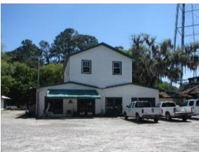
Figure 608. Mechanical Shop W-1.
