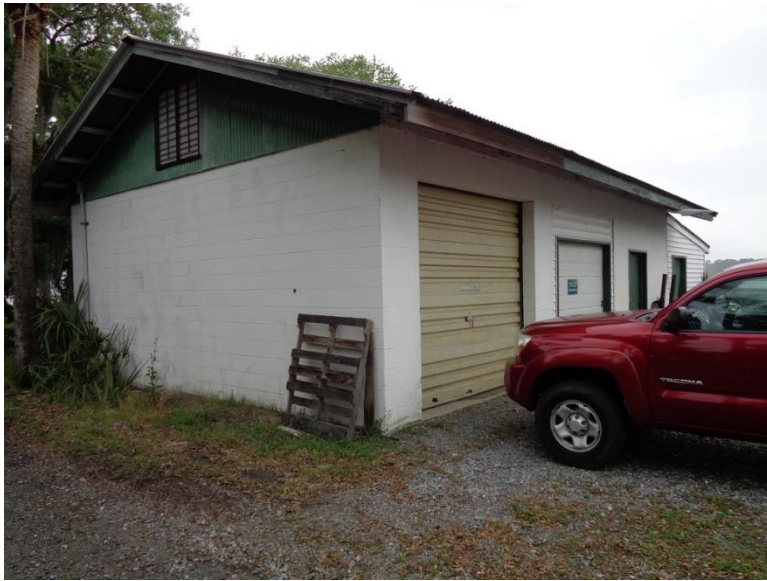
Figure 616. Marine OPS Storage Building.
