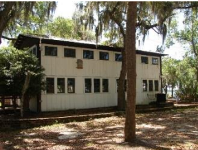
Figure 606. Mechanical Shop W-1
