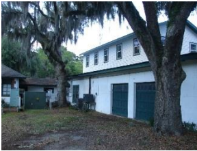
Figure 605 Mechanical Shop W-1.
