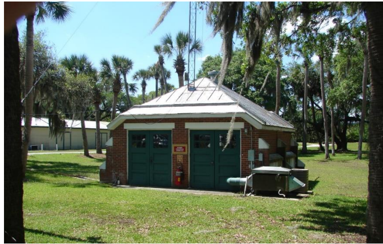
Figure 633. Chemical Storage Building.
