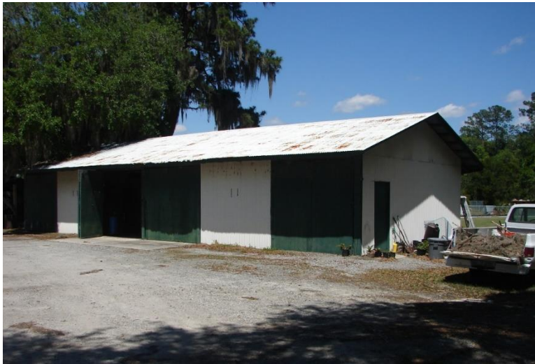
Figure 637. Maintenance Shop B.
