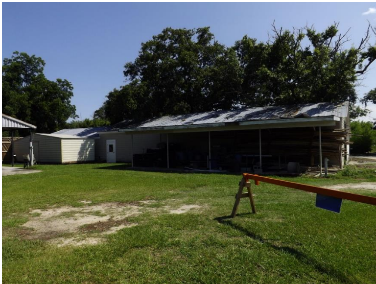
Figure 680. Storage Building No. 28.
