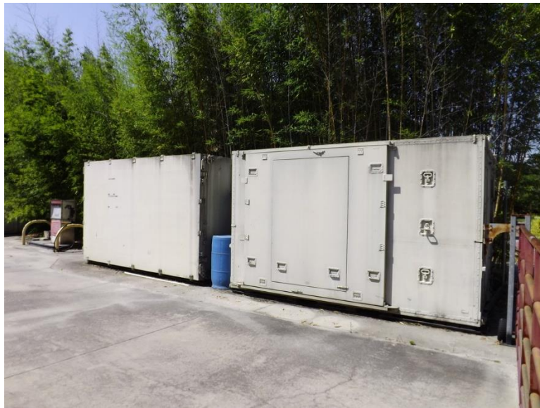
Figure 682. Storage Building No. 30.
