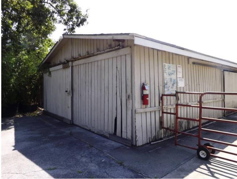
Figure 679. Storage Building No. 25.
