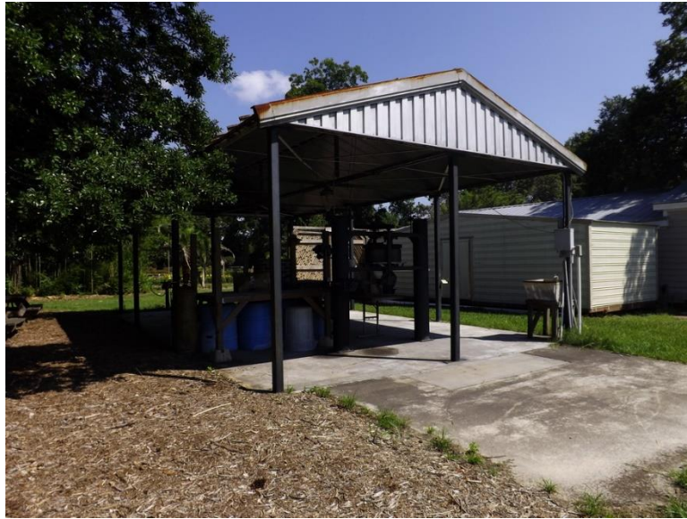
Figure 681. Storage Building No. 29.
