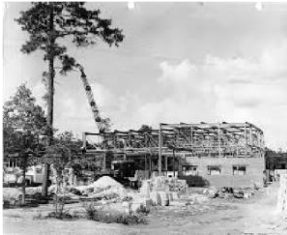
Construction of Rock Eagle 4-H Camp.
