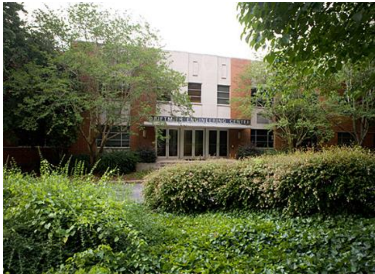
Figure 202. Driftmier Engineering Center. (Source: University of Georgia)
