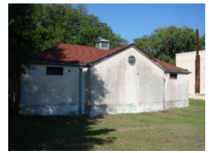
Figure 570. Fuel Storage Building.
