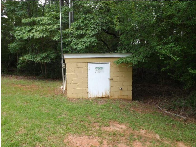
Figure 467. The pump house.
