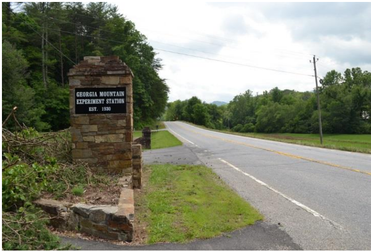
Figure 399. Stone walls and entry piers.
