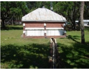
Figure 635. Chemical Storage Building.
