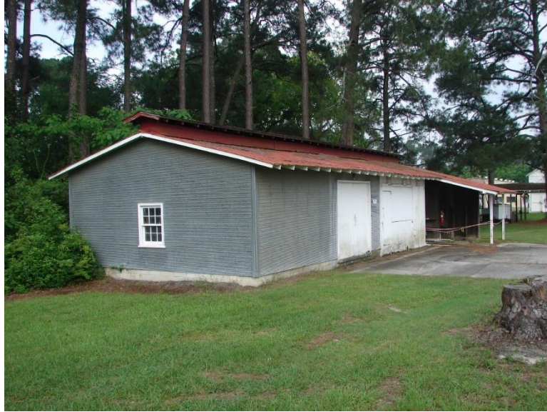
Figure 359. The Engineering Tobacco Shed.
