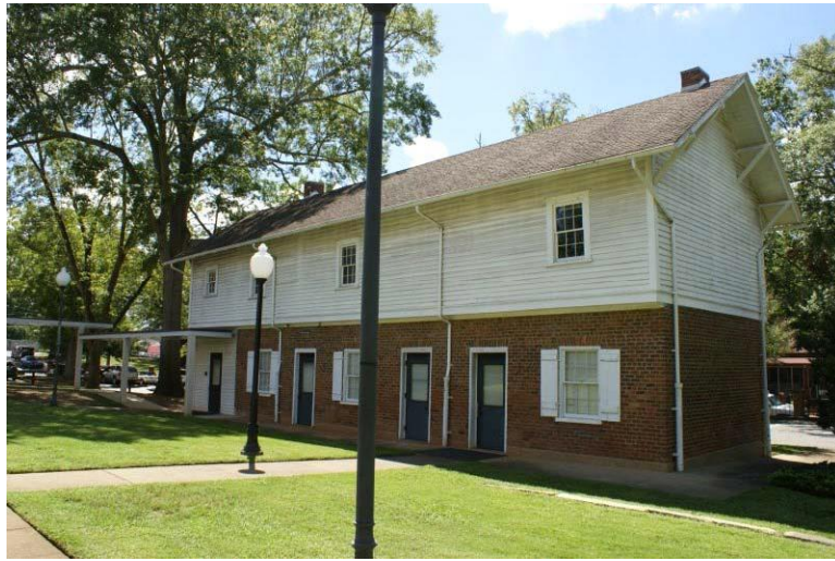
Figure 223. The carriage house, 2015.
