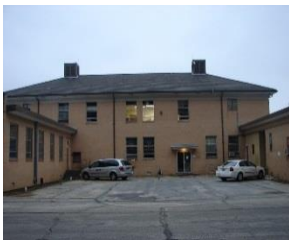
Figure 329. Rear view, Old Administration Building.
