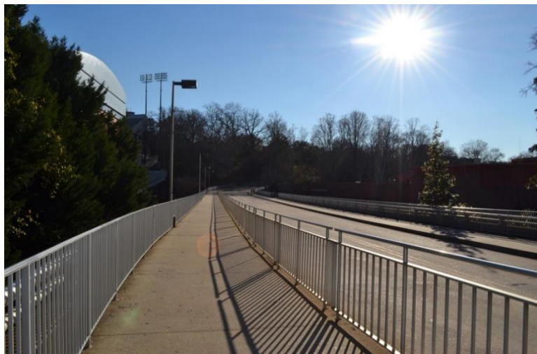
Figure 124. Jim L. Gillis, Sr. Bridge, 2015.
