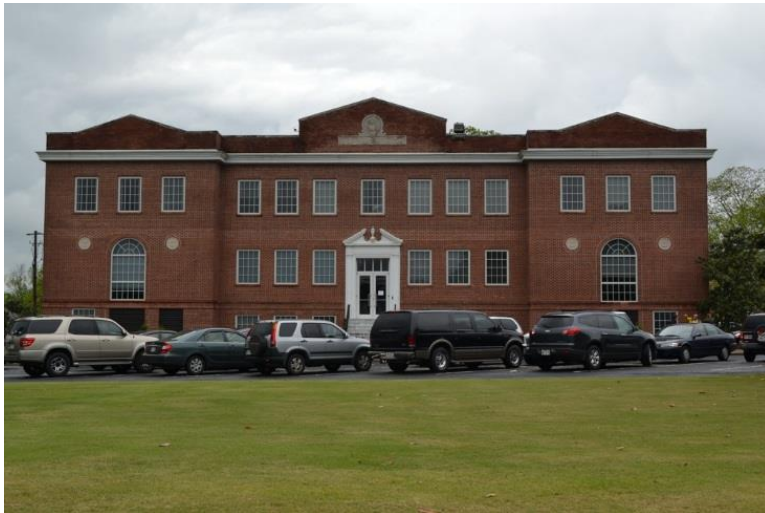
Figure 270. View toward the principal facade of Flynt, 2015.
