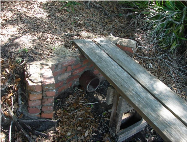
Figure 540. Brick wall and stormwater management system.
