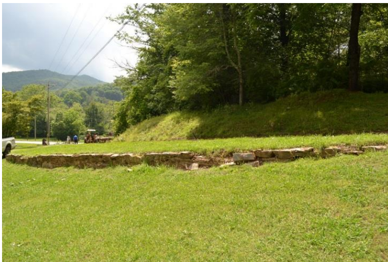
Figure 400. Entrance road retaining wall.
