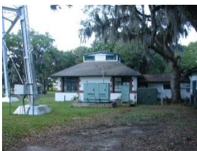
Figure 609. Mechanical Shop W-1.
