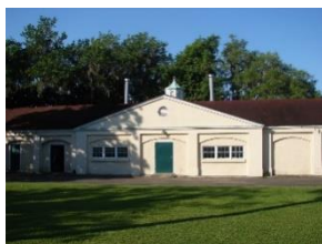
Figure 563. Maintenance and Lab Complex.
