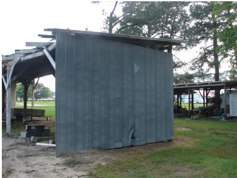
Figure 360. Ag Engineering Equipment Shed, seen far right.
