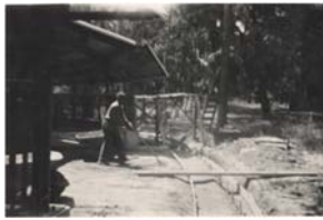
The Cattle Show Barn under construction.
