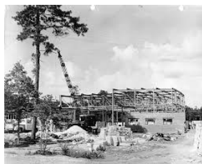
Construction of Rock Eagle 4-H Camp.
