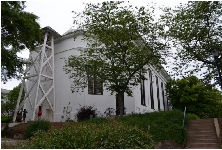
Figure 76. The bell tower, 2015.
