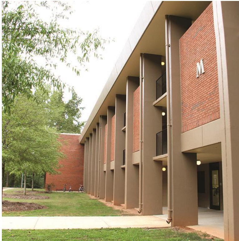
Figure 212. Rogers Road apartments. (Source: University of Georgia)
