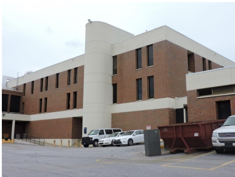
Figure 197. Veterinary School complex, 2015.
