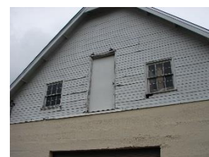
Figure 275. Detail of Mule Barn gable, 2015.
