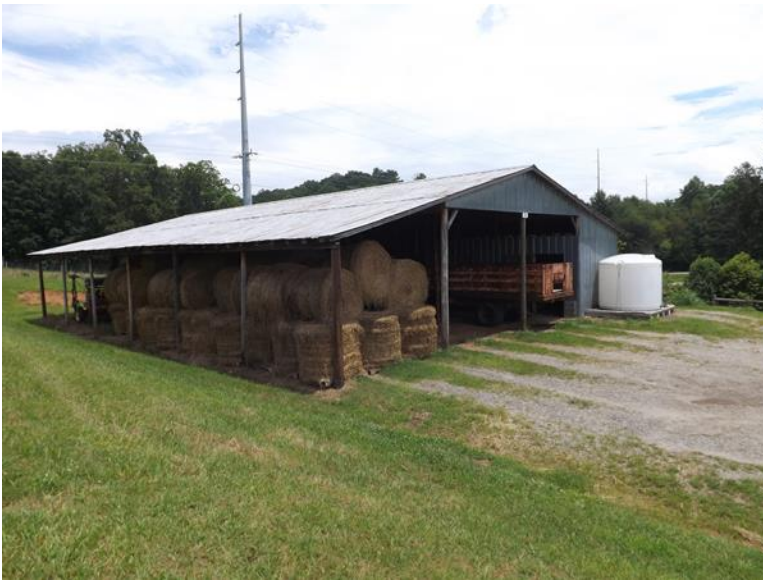
Figure 407. The feed barn.
