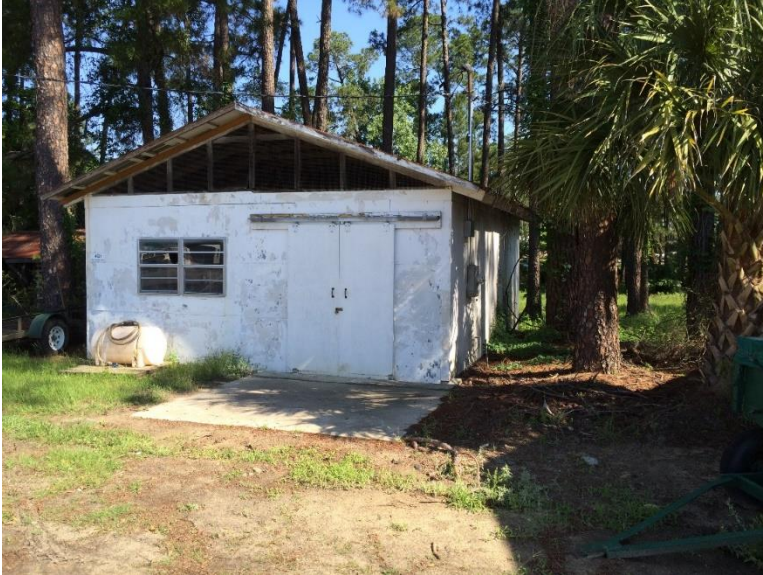
Figure 367. The Plant Pathology Growth Chamber.
