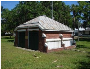
Figure 634. Chemical Storage Building.
