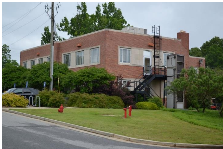
Figure 273. View northwest toward the Cowart Building, 2015.
