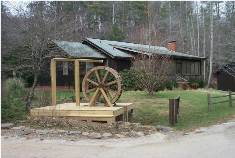
Figure 476. Manager's House/Director's House/Caretaker's House, with water wheel in foreground. (Source: University of Georgia Office of University Architects)
