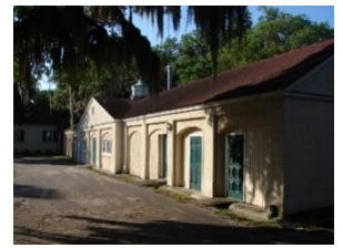
Figure 564. Maintenance and Lab Complex.
