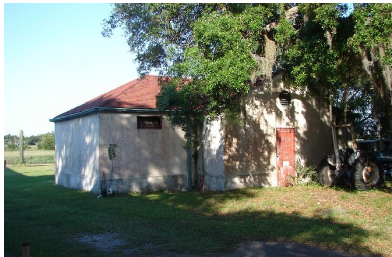
Figure 569. Fuel Storage Building.
