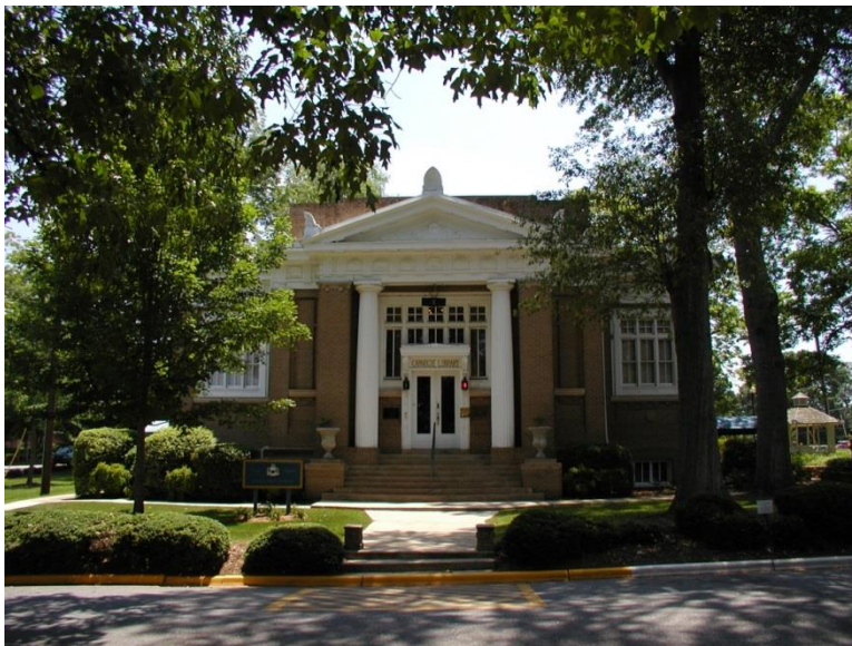
Figure 243. Carnegie Library. (Source: Historic Buildings Preservation Plan)
