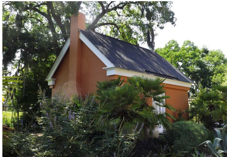
Figure 661. Superintendent's Office, built circa 1919, later Office 15, and now the Bridal Cottage at the Mediterranean Garden. (Source: Coastal Georgia Botanical Gardens, 2013)
