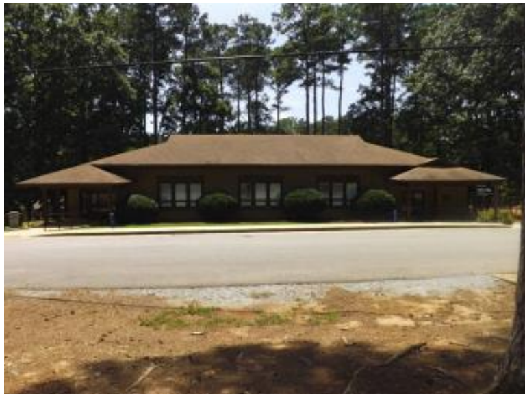
Figure 453. The Callaway Building.
