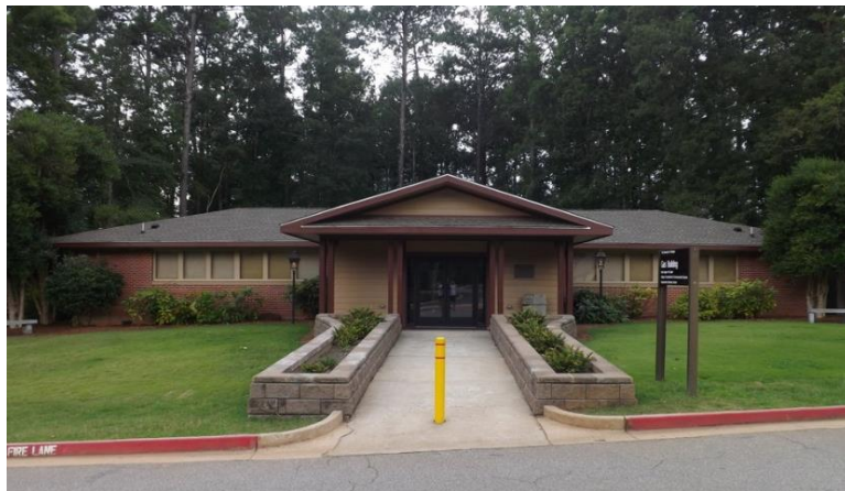
Figure 457. L.P. Gas Building.
