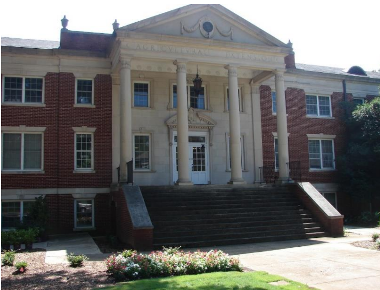
Figure 183. Hoke Smith Building, 2015.
