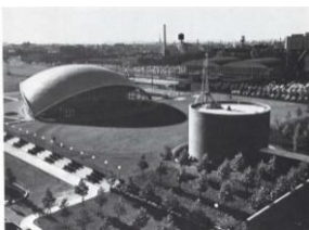
Figure 41. Kresge Auditorium and Chapel, Massachusetts Institute of Technology, Cambridge. (Source: Turner, 261)
