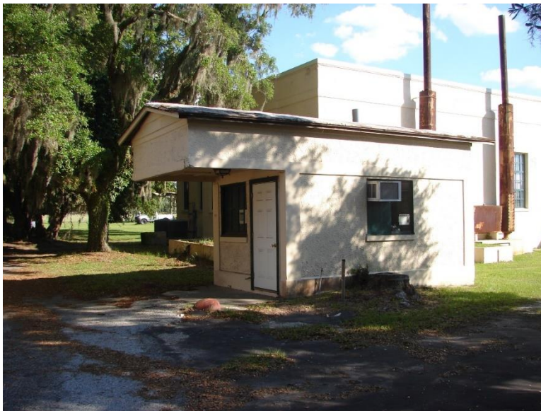
Figure 565. South End Filling Station.
