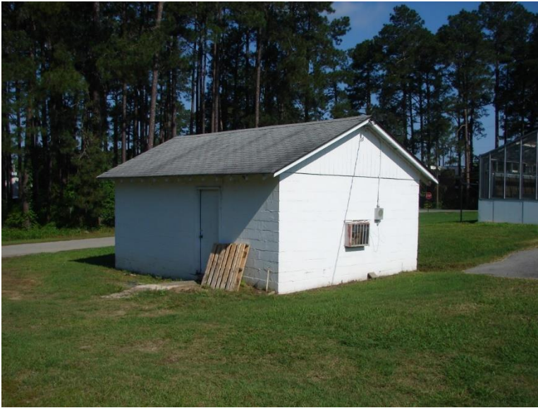
Figure 364. ARS Storage Building.
