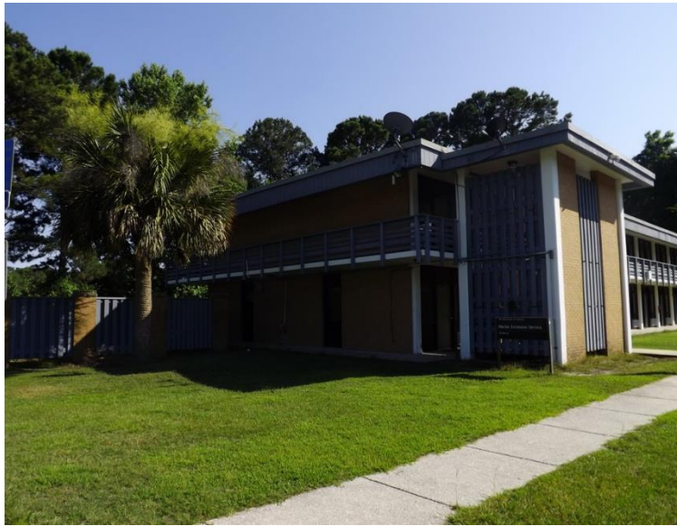
Figure 647. UGA MAREX Dormitory.
