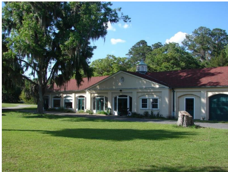
Figure 562. Maintenance and Lab Complex.
