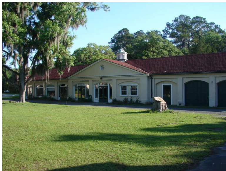
Figure 558. South End Office Building.
