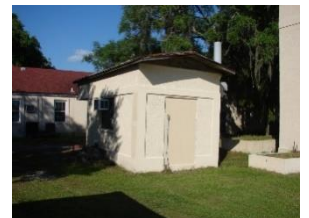
Figure 566. South End Filling Station.
