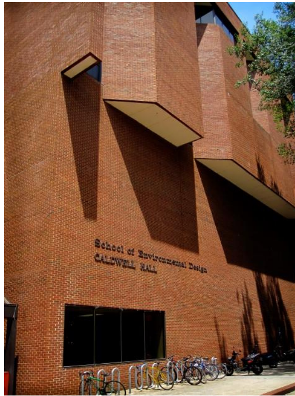
Figure 43. Caldwell Hall (UGA.46). (Source: University of Georgia)
