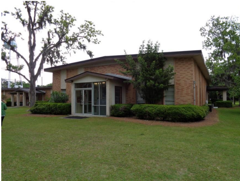
Figure 604. Principal facade of the Roebing Lab.
