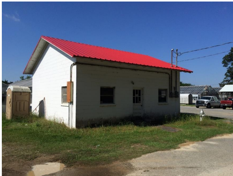
Figure 369. The Grass Br Headhouse and Greenhouse.
