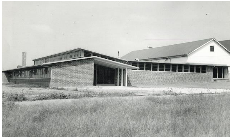
Figure 283. The Food Processing Plant annex during construction in 1952 (Source: University of Georgia).
