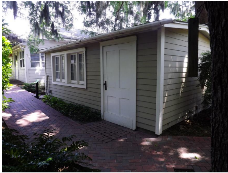
Figure 677. Laundry Building No. 18.
