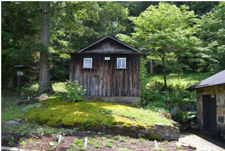
Figure 398. The tool storage shed, which is located east of the work center/storage building.
