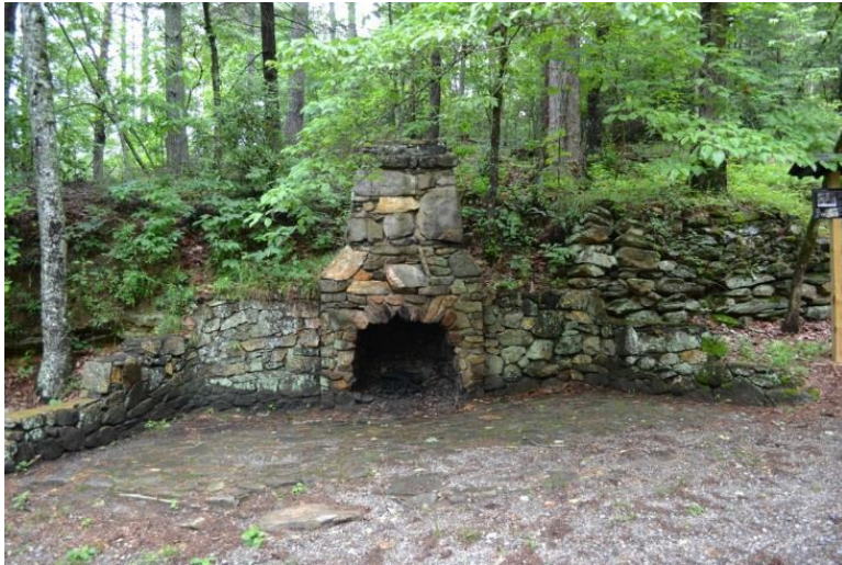
Figure 424. Stone fireplace west of the storage shed.
