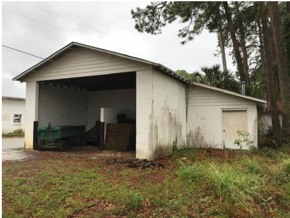
Figure 378. Soil Sterilizer Shed. (Source: University of Georgia)
