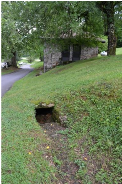
Figure 403. The stormwater management system that parallels Georgia Mountain Experiment Station Road near the Office and Seed Lab.
