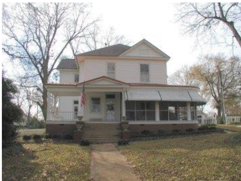
Figure 238. Former President's Cottage. (Source: Historic Buildings Preservation Plan)
