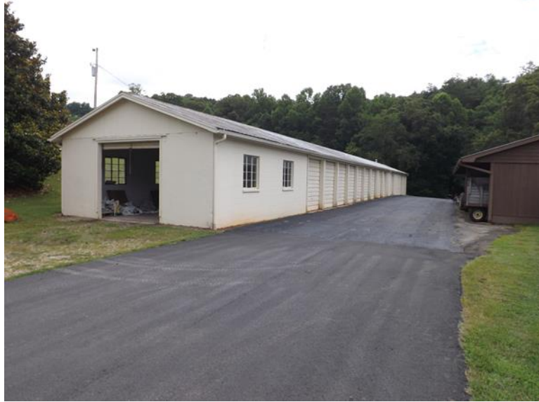
Figure 409. The utility warehouse.
