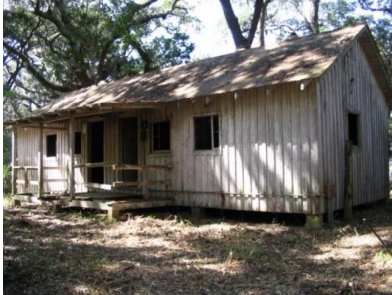
Figure 652. Skidaway Interpretive Cabin.
