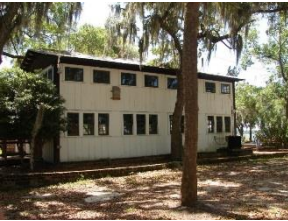
Figure 606. Mechanical Shop W-1
