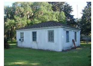
Figure 519. Azalea Apartment, rear and side view.
