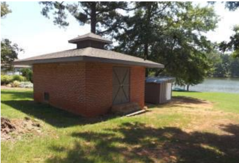
Figure 464. Pool 1 Filter House.
