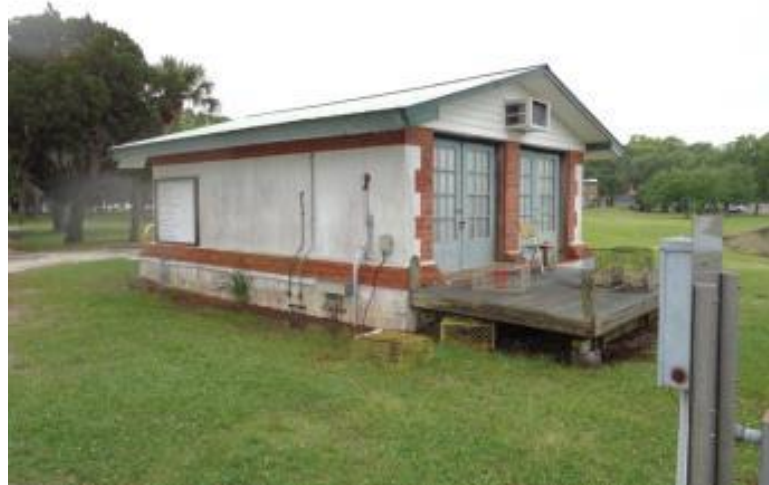
Figure 636. Fuel Oil Storage.
