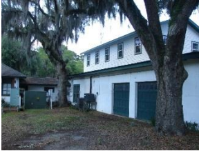
Figure 605 Mechanical Shop W-1.
