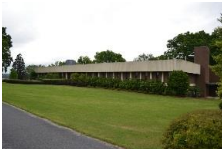
Figure 306. View southwest toward the Redding Building, 2015.
