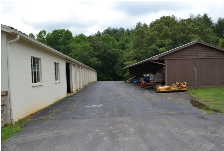
Figure 411. The maintenance vehicle shed.
