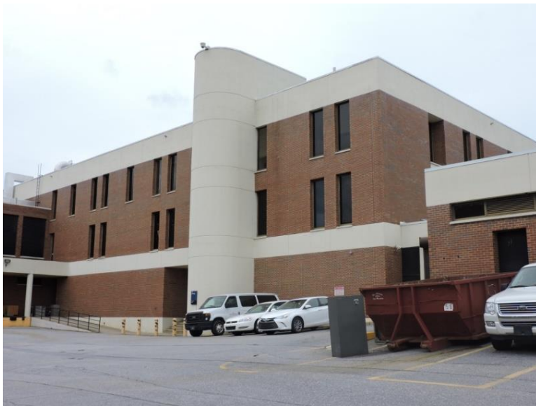
Figure 197. Veterinary School complex, 2015.
