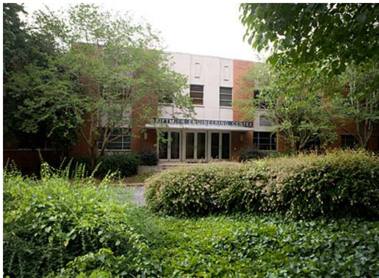
Figure 202. Driftmier Engineering Center. (Source: University of Georgia)
