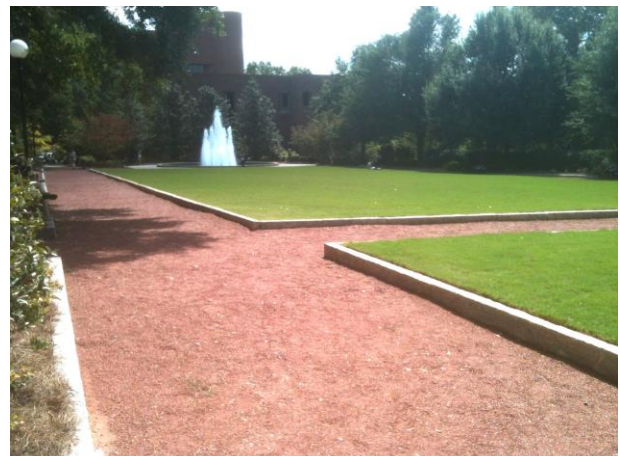
Granular Paving – Herty Field
