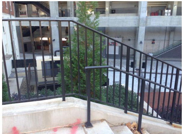
Handrails & Adjacent Guardrail – Reed Plaza
