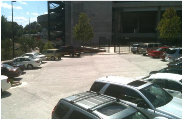
Porous Paving Parking Lot – Reed Plaza
