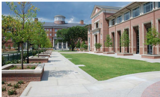
Green Roof – Tate Student Center
