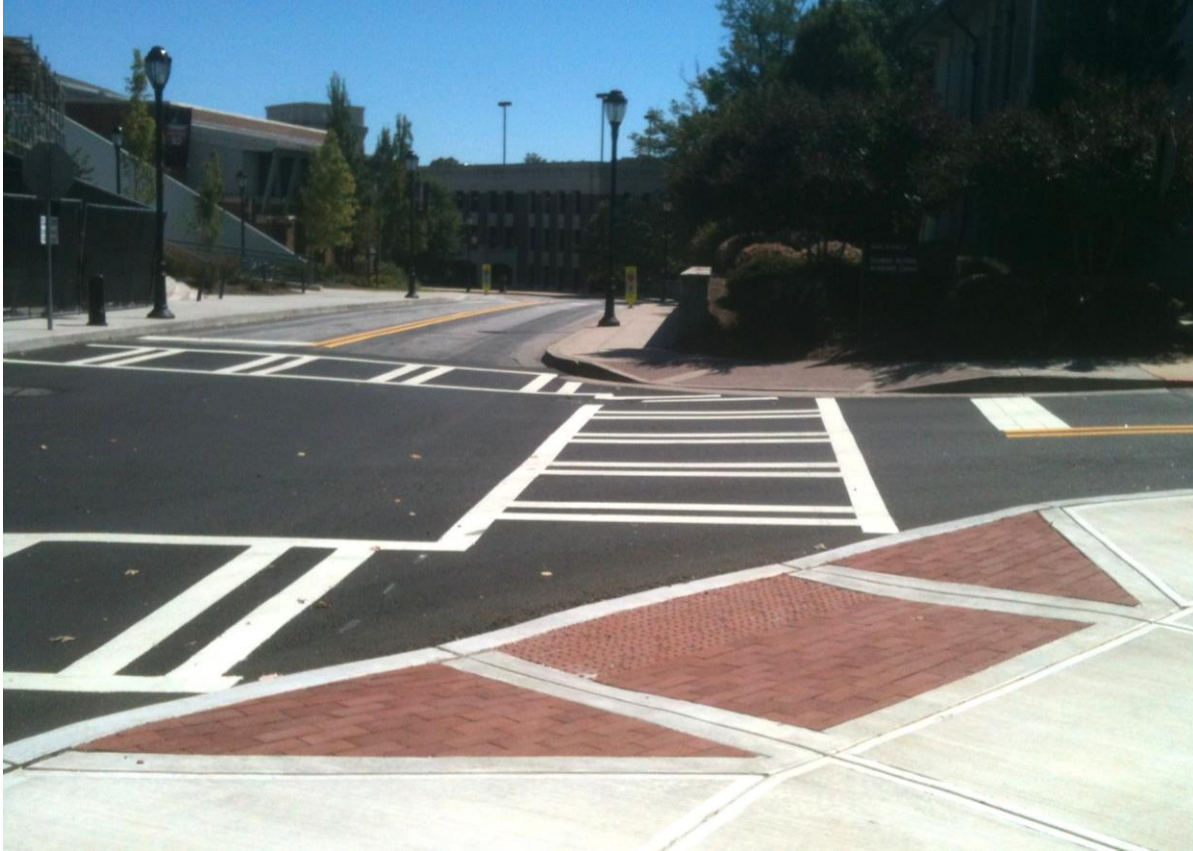
Crosswalks and Curb Cut with Truncated Domes – Stegeman Coliseum
