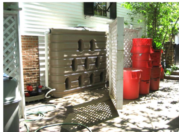
Above-Ground Cistern – Founders House
